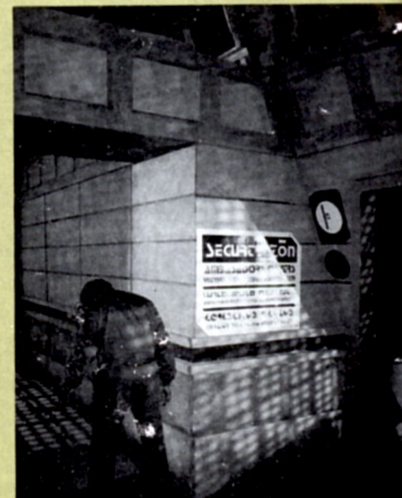
The corridor to customs and the station's secure zone, part of Stage B.
